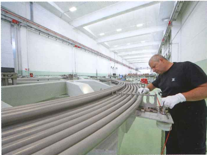
Technician checking the tooling used for the winding of the conductor for the ITER Toroidal Field coils, ASG Superconductors, La Spezia, Italy
